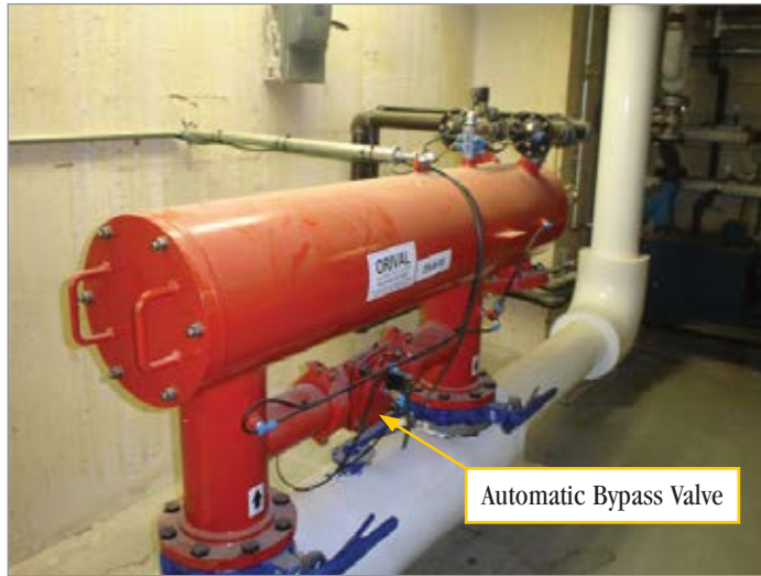
Figure 1: Filter Installation
