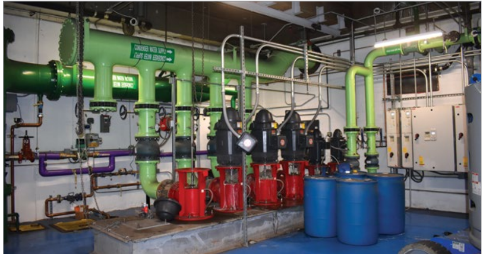
The pumping system distributes chilled water at the Norman plant.
