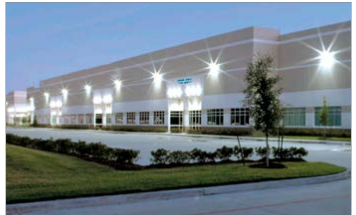
EvapTech Gulf Services building
