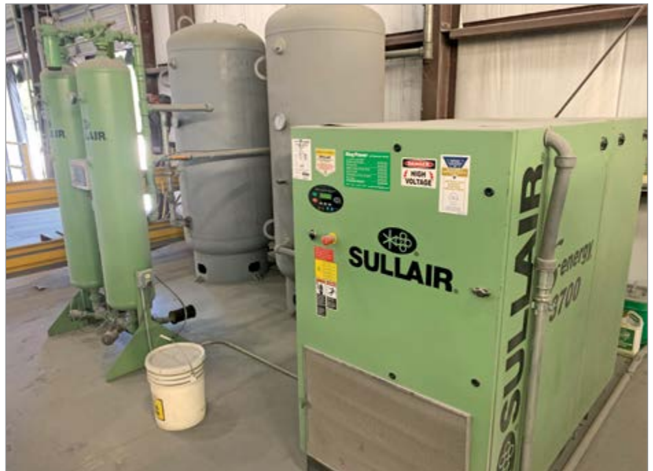
A company manufacturing tile and flooring installation systems relies on this oil-flooded rotary screw air compressor and heatless desiccant compressed air dryer.
