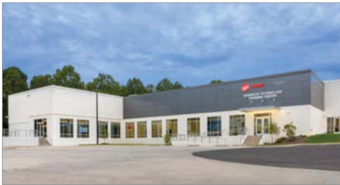
The Trane Advanced Technology Training Center in Davidson, NC
