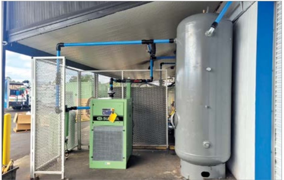
This customer has a variable-speed, oil-flooded, rotary screw air compressor located inside its facility to protect it from the Florida humidity, and an 800 cfm, non-cycling, refrigerated compressed air dryer under an enclosure.
