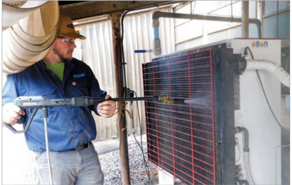
A technician pressure washes the heat exchanger on an oil-flooded, rotary screw air compressor.
