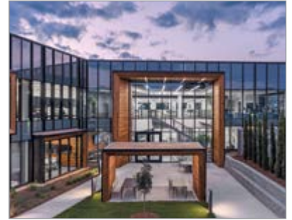
Boehringer Ingelheim Animal Health facility in Athens, GA (Photo credit: Cory Klein of Cory Klein Photography & CKP Studio ©2024)
