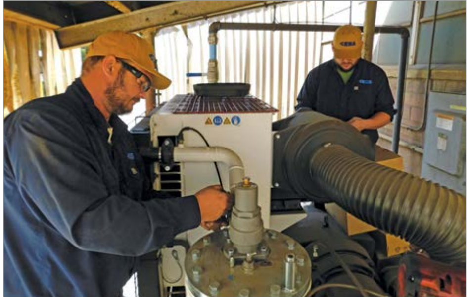
A technician performs a scheduled preventive maintenance service on an oil-flooded, rotary screw air compressor at J.C. Steele & Sons.
