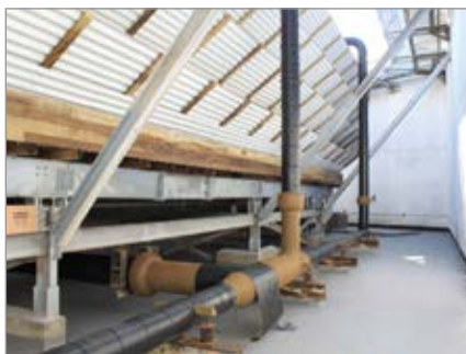
Overview of the complete Denso corrosion protection system for cooling towers for pipes, valves and fittings.
