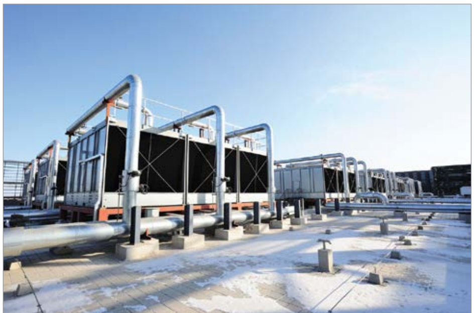
Evaporative cooling towers are an integral part of many data center cooling systems, depending on their location.
