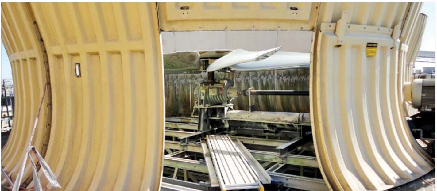
Gearboxes are used as speed reducers to slow the rotational speed from the incoming motor to the outgoing fan of a cooling tower.
