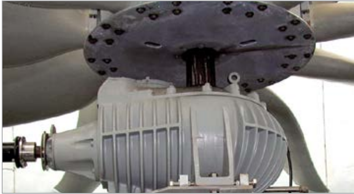
To address high operating temperatures, select a gear drive with integral “cooling fins” designed into the housing.
