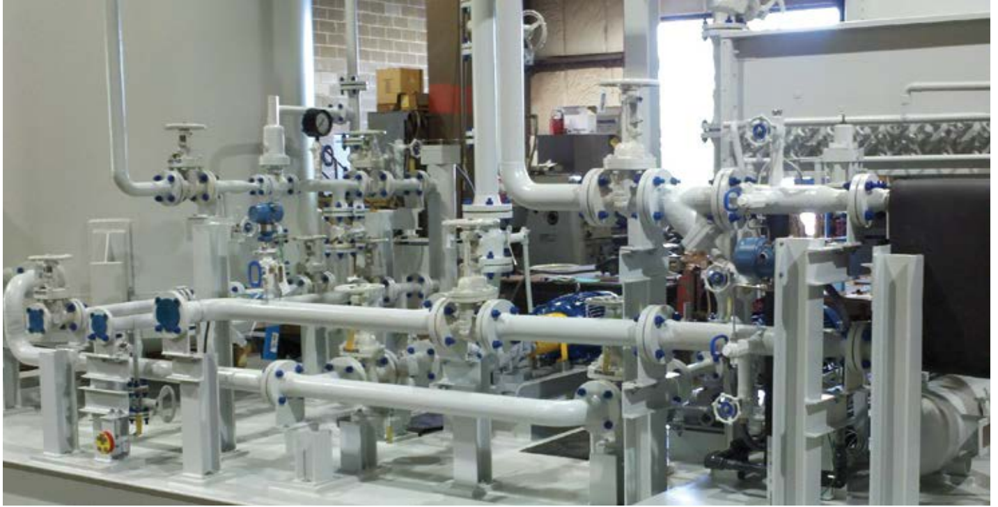
There are bypass valves around the chiller, pumps, ultraviolet sterilizing equipment and other components - so maintenance can be done.
