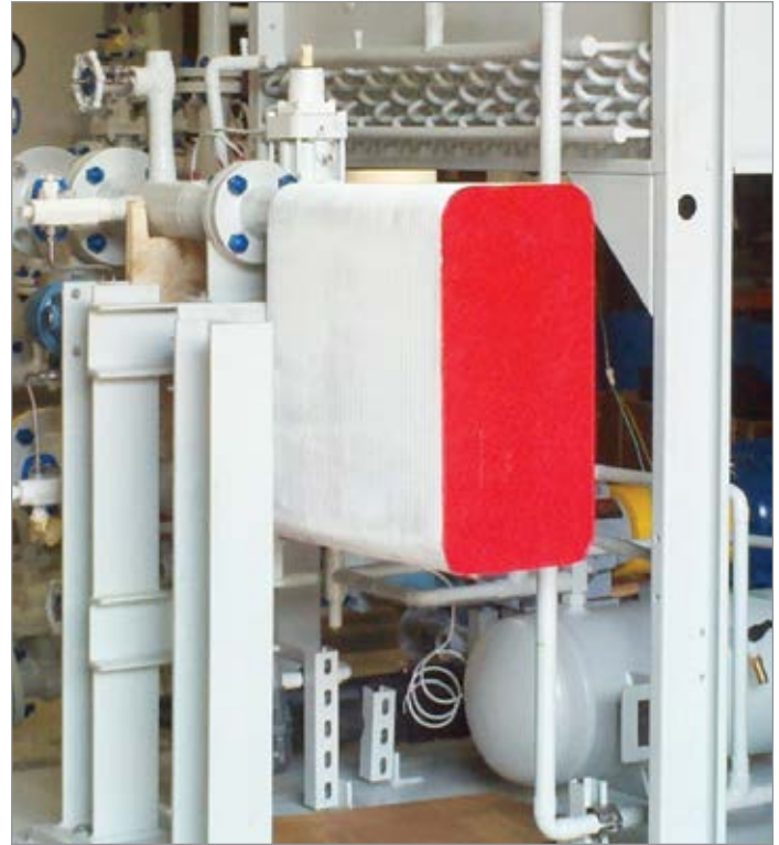
Very high efficiency evaporators used with double wall laser welded plates to isolate refrigerant from potable water.
