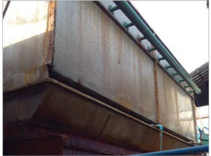
Figure 4. The evaporative condenser at the plant.
