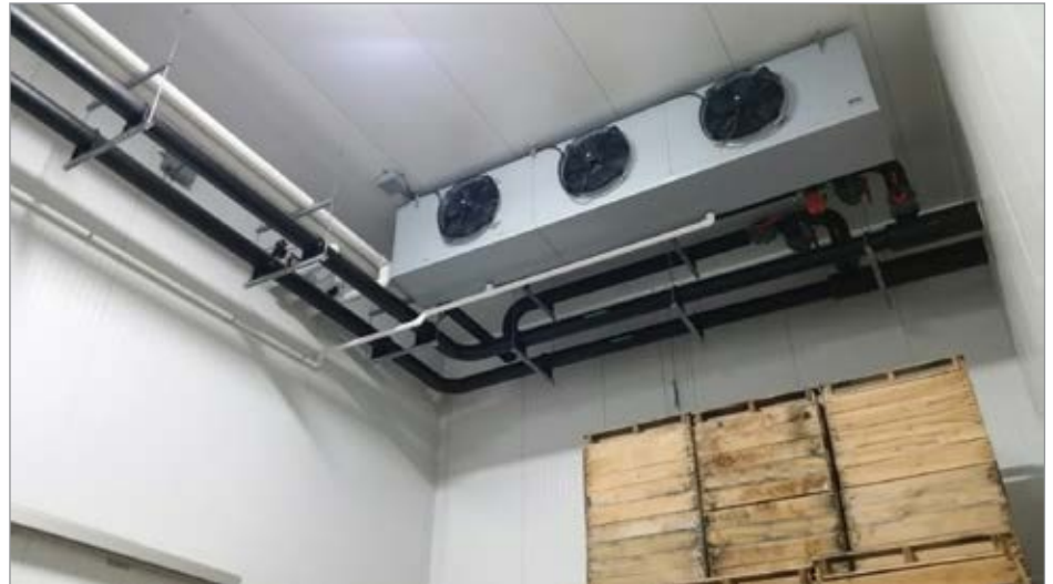
The COOL-FIT ABS Plus is designed for conveying water-based coolants with temperatures from -58°F to 104°F (-50°C to +40°C).
