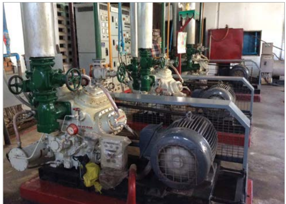
Figure 2. The refrigeration plant is a two stage, closed intercooler ammonia (R717) system consisting of three reciprocating compressors of the brand MYCOM – first in the image C1 (50 HP), C2 (50 HP) and C3 (75 HP).
