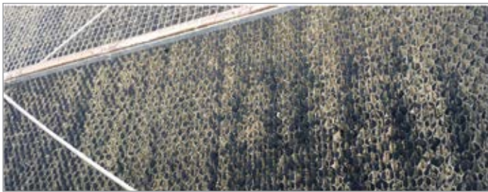
Cooling tower fill media exhibiting severe scaling, before UET treatment.
