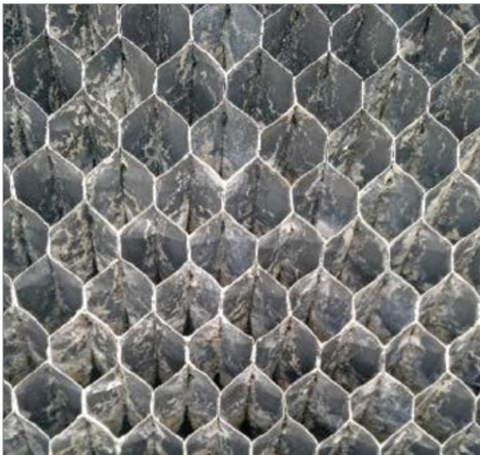
Cooling tower fill media free of scaling, after UET treatment.
