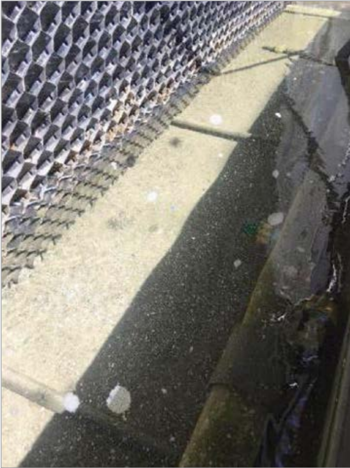
Cooling tower cold-water basin free of scaling and biological growth, after UET treatment.
