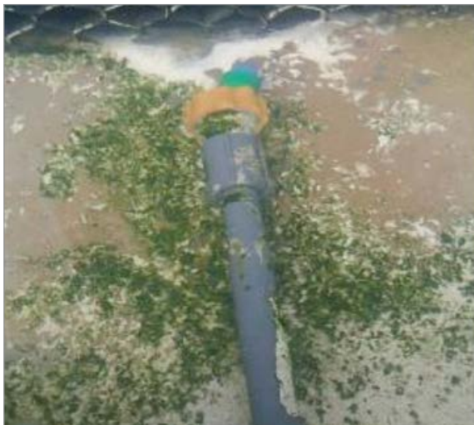
Cooling tower cold-water basin exhibiting scaling and biological growth, before UET treatment.
