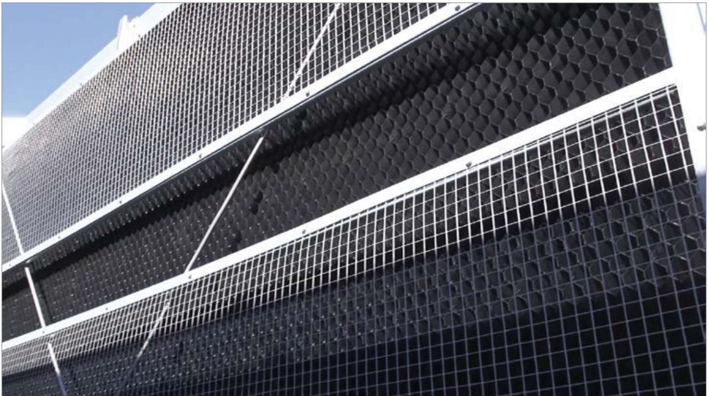
An air inlet screen helps qualify a cooling tower as FM APPROVED, because in the event of a fire, it keeps fill materials and debris contained within.
