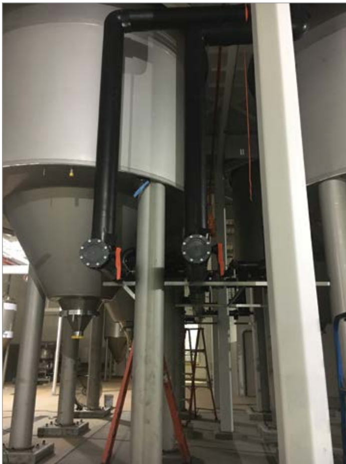
Shown is one of 16 new 60-foot tanks in the Bay 7 Loop Project. The expansion included a run of 1,000 feet of COOL-FIT piping to convey chilled water to keep the beer tanks cold.
