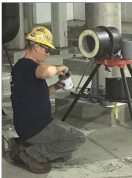
COOL-FIT is easily joined using cement and a flat brush. Pictured is Mike Sharp, Leadman for M. Davis & Sons, Inc., the Delaware-based contractor most heavily involved with the COOL-FIT installation at Dogfish Head.
