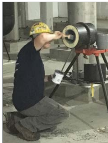
COOL-FIT is easily joined using cement and a flat brush. Pictured is Mike Sharp, Leadman for M. Davis & Sons, Inc., the Delaware-based contractor most heavily involved with the COOL-FIT installation at Dogfish Head.
