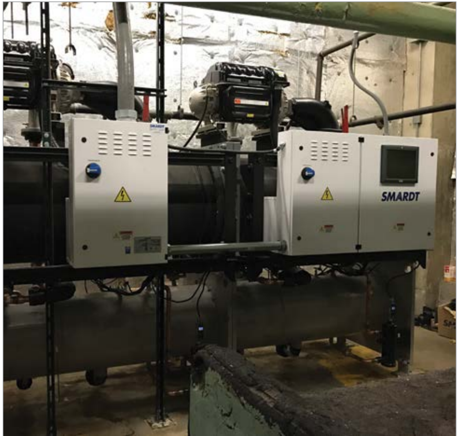
The upgraded installation at RUMC includes a new 300-ton chiller with two 150-ton compressors.
