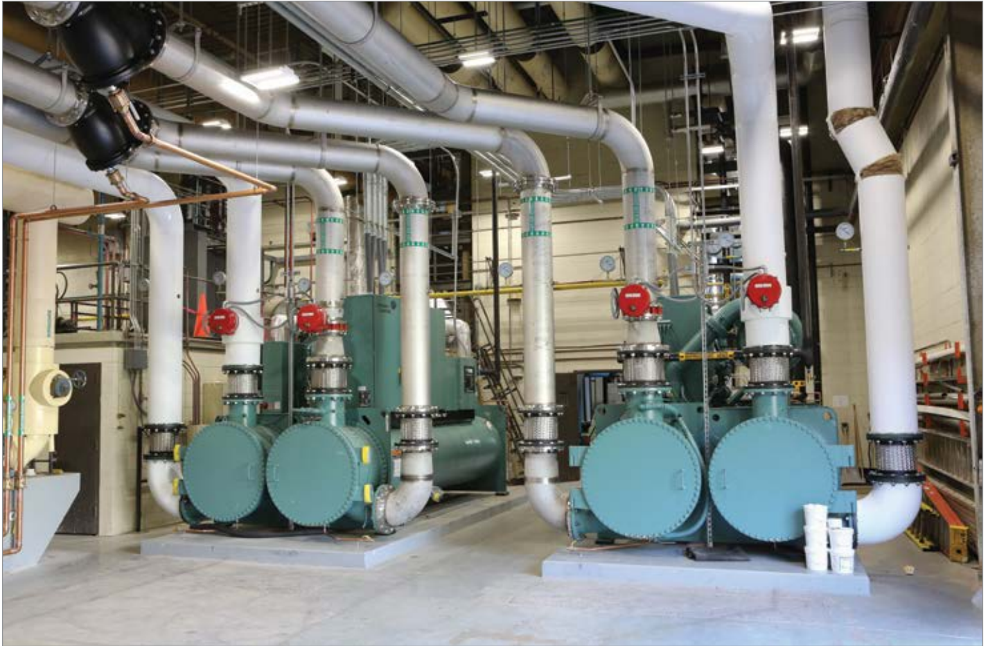
Magnetic-bearing centrifugal chillers at the central chiller plant.
