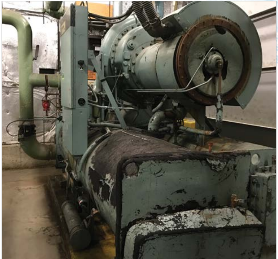
RUMC replaced two aging fixed-speed 300-ton water-cooled centrifugal chillers (shown here) with energy-efficient Smardt split-shell chillers with Danfoss Turbocor compressors, reducing installation costs and saving $75,000 in annual operating costs.
