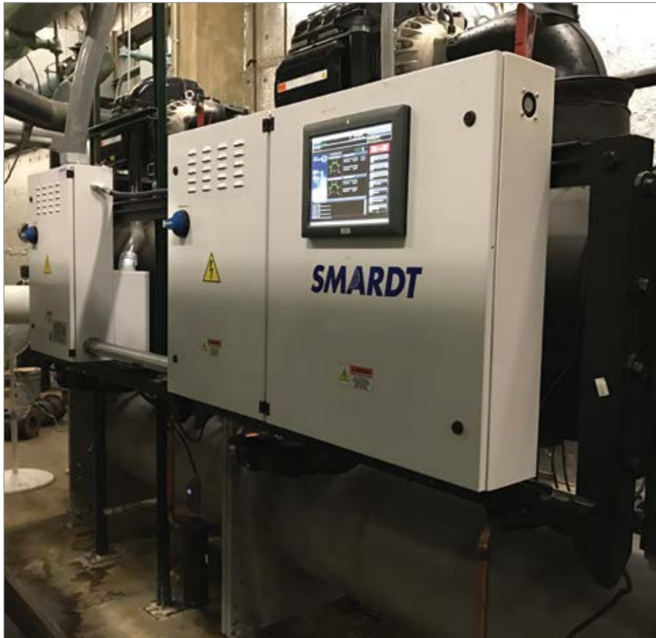
The new compressor's user-friendly control system interfaces with the chiller controller, helping simplify system configuration and commissioning.
