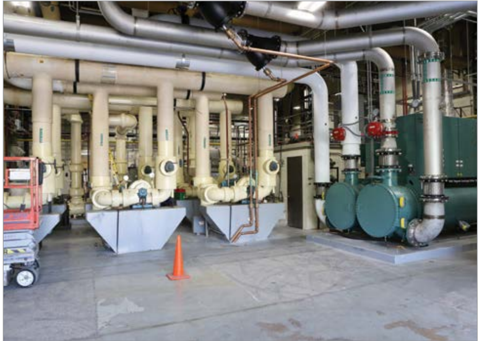
The medical center’s central chiller plant leverages pumps with VSDs (center) to achieve energy efficiencies.
