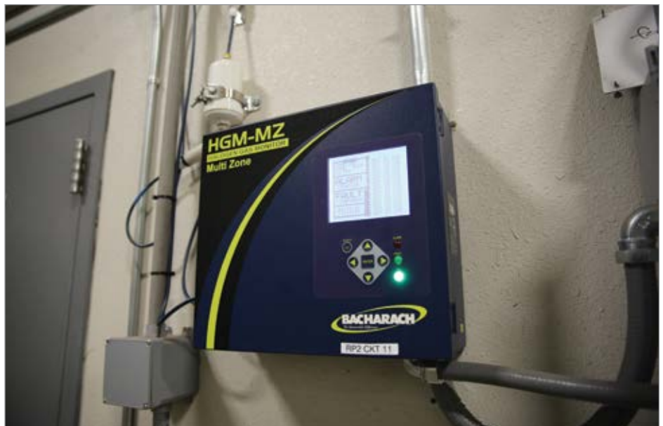
As a reliable refrigerant monitor, Bacharach's HGM-MZ ensures Xcel Energy chillers remain in good operating condition.
