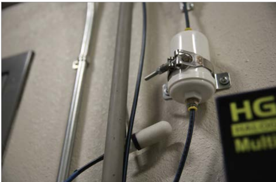
Shown is a charcoal filter and detection point beside the HGM-MZ refrigerant monitor.
