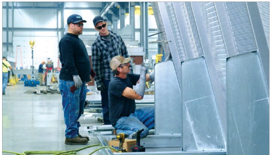
Assembly of an eco-Air Series Dry Cooler in the Key Building located at EVAPCO headquarters in Taneytown, MD.
