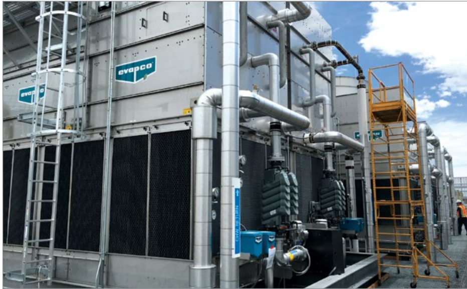
An EVAPCO eco-ATWB-H fluid cooler
