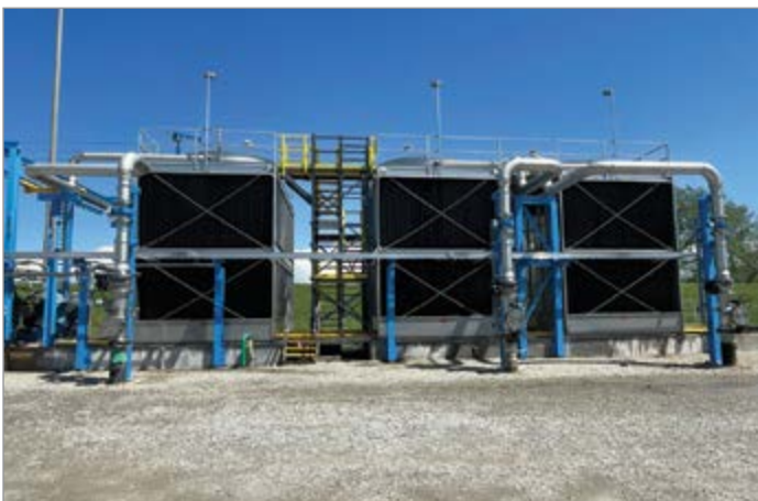
Midwest Machinery engineered a three-cell, double-stack, dual air inlet, crossflow, factory-assembled Marley cooling tower on the old cooling tower's foundation.
