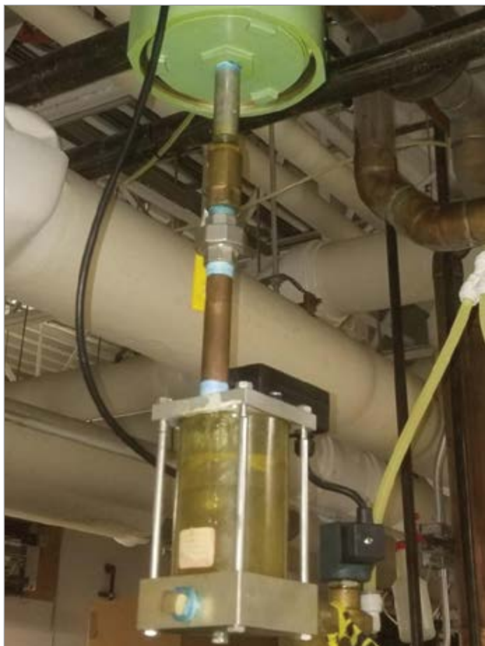
The refrigerated compressed air dryer pre-filter was the next possible trouble spot.
