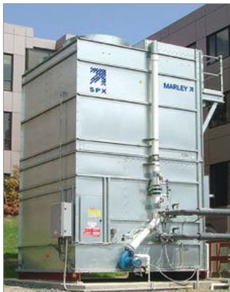
Fluid cooler cooling towers combine closed-loop cooling and evaporative heat rejection in a single, unified package.
