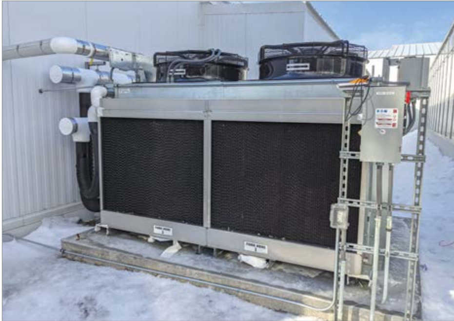
A New England-based automotive plastic interior parts manufacturer needed five 34-ton adiabatic fluid coolers, each sized for 81.3 gpm, with an entering temperature of 95°F (35°C) and a leaving temperature of 85°F (29°C).
