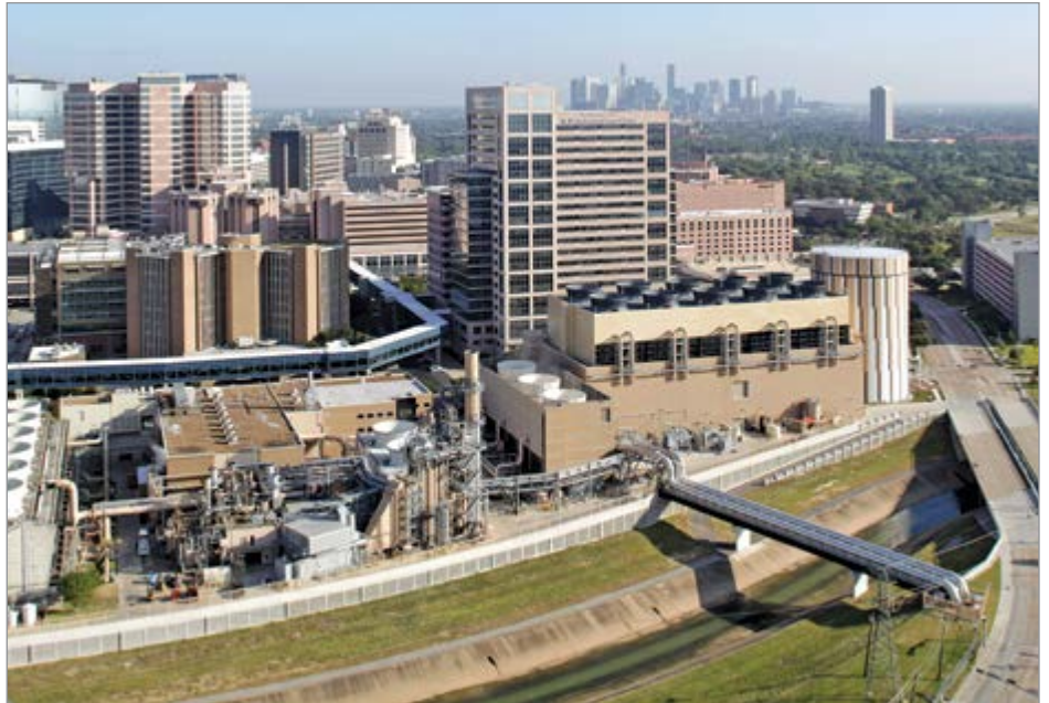
Burns & McDonnell provided engineering, procurement and construction for the $377 million expansion of a district energy plant in the South that included an 8.8 million-gallon chilled water thermal storage tank and a new plant with four 8,000-ton electric drive chillers. (Photo: Paul Howell)
