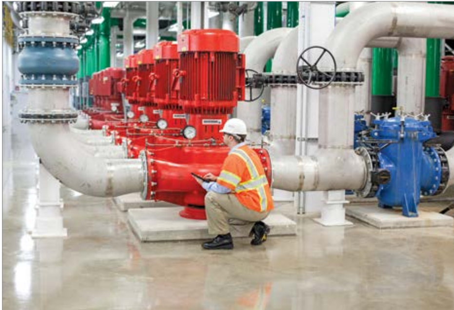
Burns & McDonnell added a new plant building with two 2,650-ton chillers, five cooling towers and primary/secondary pumping for a chilled water plant for a healthcare client in the Midwest. (Photo: Michael Robinson)
