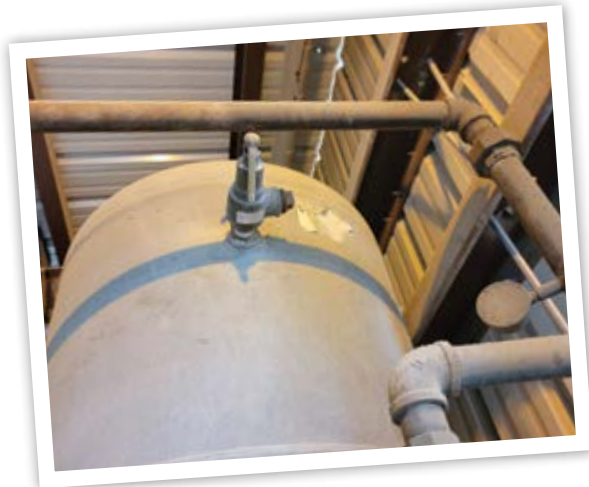
Plugging this dry tank's safety valve was a poor way to stop a leak.
