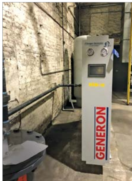
Installing the nitrogen generator
