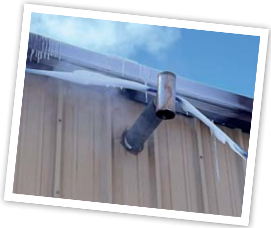
A 37°F (3°C) pressure dew point isn't low enough when the ambient temperature reaches -15°F (-26°C).
