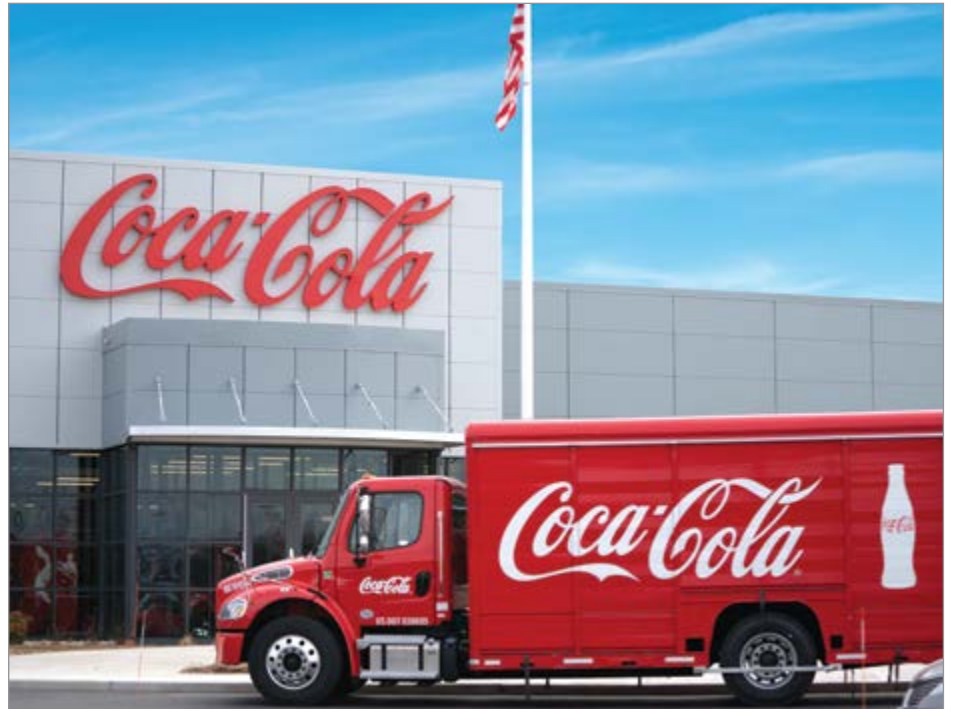
Coca-Cola Beverages Northeast is located in South Windsor, CT.
