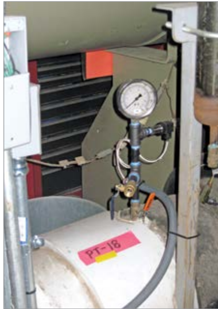
This single pressure sensor installation includes a manual blowdown port and gauge.
