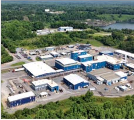
Albemarle Corporation's plant in Kings Mountain, NC
