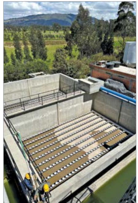
A diffuser installation in Colombia using advanced membrane materials.
