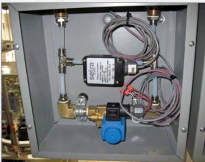
This ISG packaged DP sensor assembly includes automatic blowdown.
