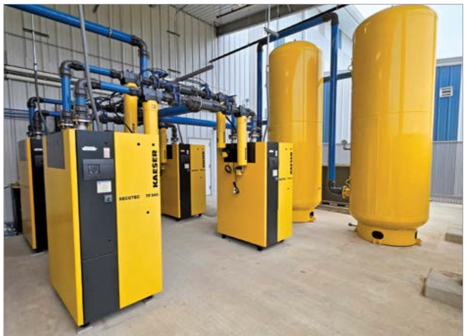
The recycling plant’s compressed air system includes full redundancy.
