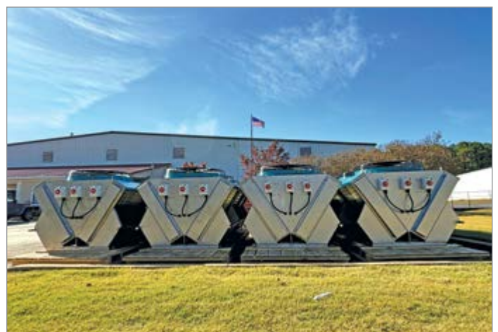
Adiabatic coolers featuring motor disconnect switches for on-site controls integration
