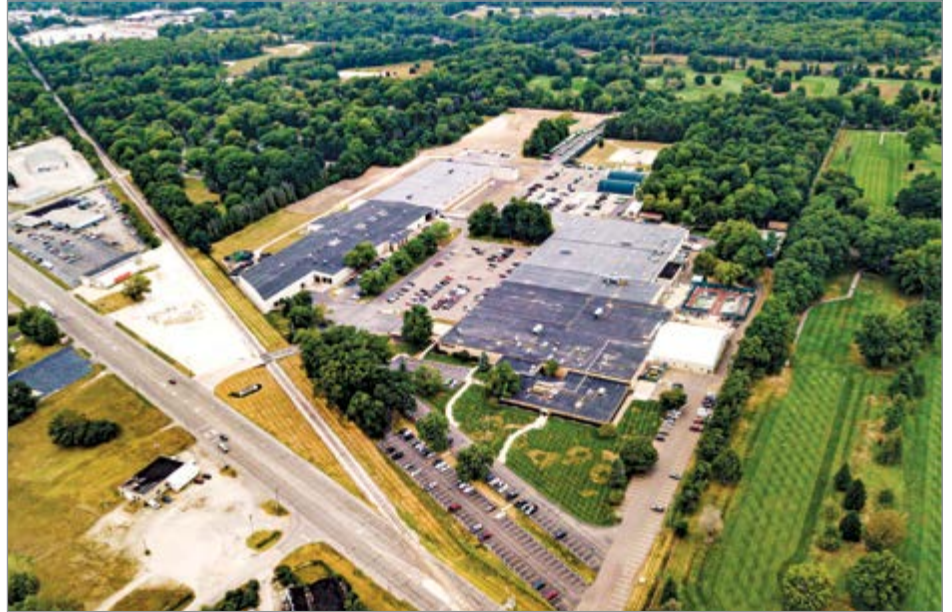
The Sullair manufacturing campus in Michigan City, IN
