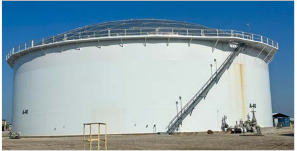
The five-million-gallon collection basin.
