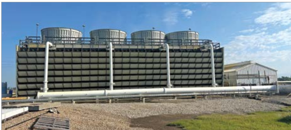
The refinery's largest cooling tower cools 35,000 gpm.
