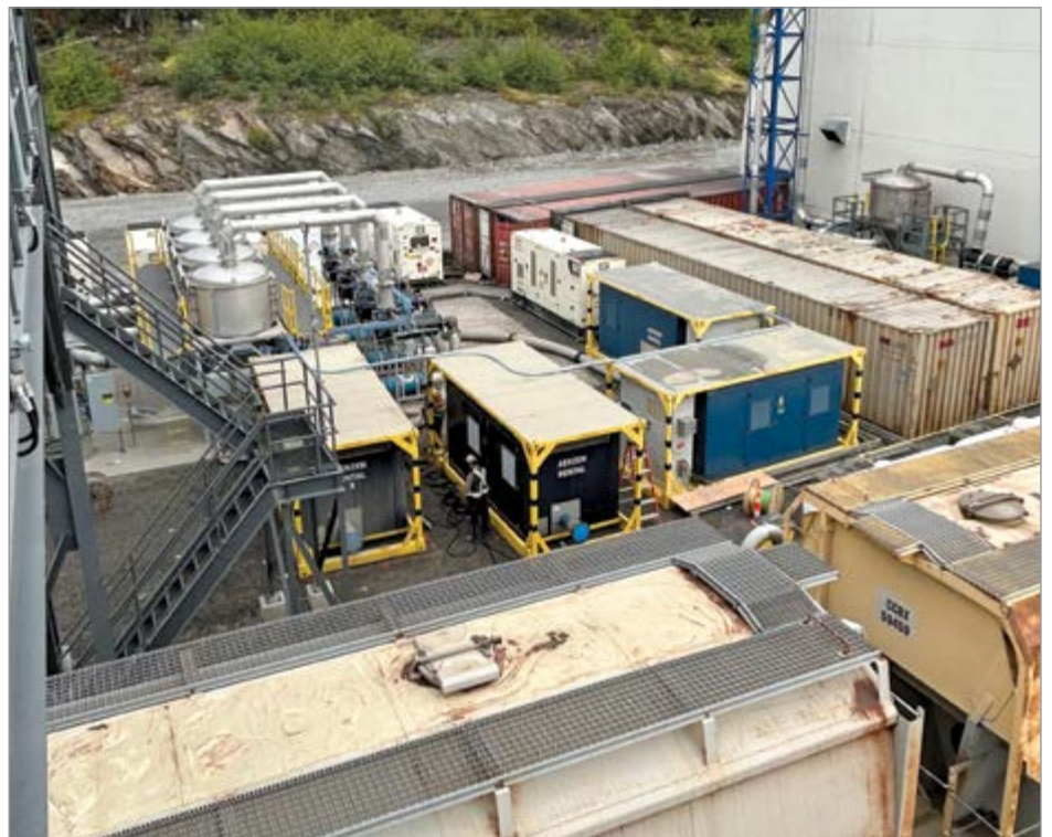
These vacuum blowers were rented while permanently installed vacuum blowers were on order.
