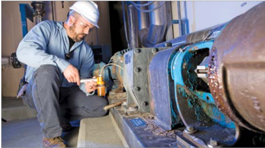
Consistently use correct sampling techniques for the best lubricant maintenance recommendations. (Photo: Noria)
