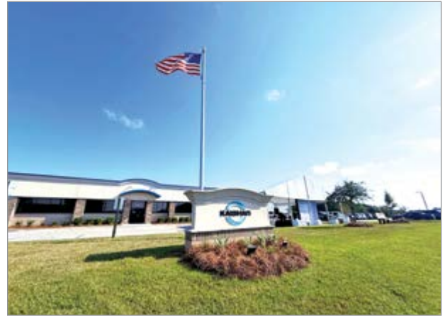
Kaishan Compressor USA’s headquarters in Loxley, AL
