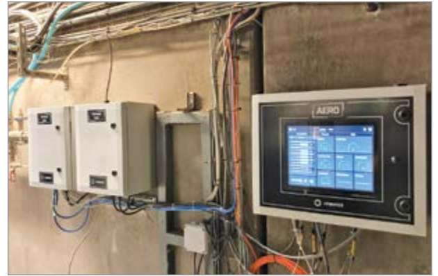
This controller is the heart of the monitoring network. Its 12-inch color display offers full system visibility in real time.
