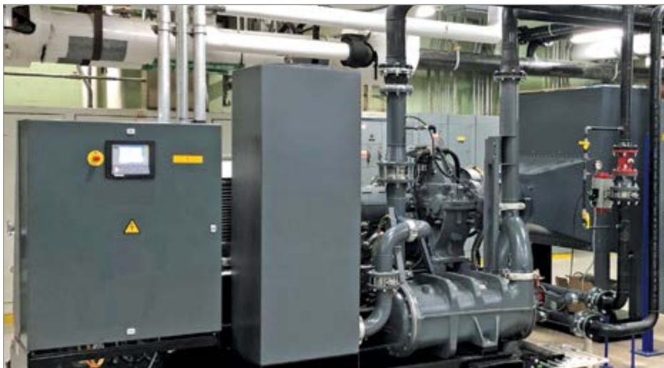
Advanced microprocessor controls (shown at the top left) minimize surge events
