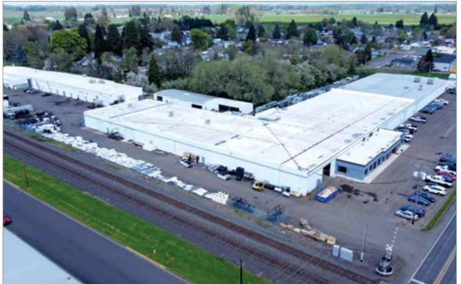
G&D Chillers headquarters in Junction City, OR
