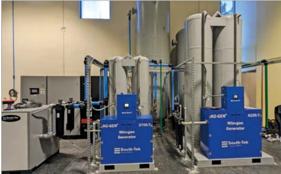
The project included two nitrogen generators supported by an integrated system of an air compressor, a refrigerated compressed air dryer, filtration, storage tanks and control and performance monitoring tools.
