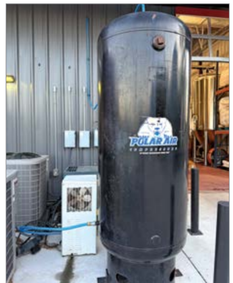
The brewery's oil-injected, air-cooled, rotary screw air compressor is located outside under an awning. Compressed air feeds into a noncycling refrigerated compressed air dryer, then a dry storage tank.
