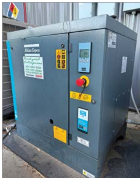
The brewery's oil-injected, air-cooled, rotary screw air compressor is located outside under an awning. Compressed air feeds into a noncycling refrigerated compressed air dryer, then a dry storage tank.
