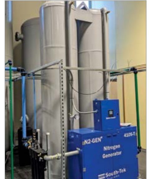
The project included two nitrogen generators supported by an integrated system of an air compressor, a refrigerated compressed air dryer, filtration, storage tanks and control and performance monitoring tools.
