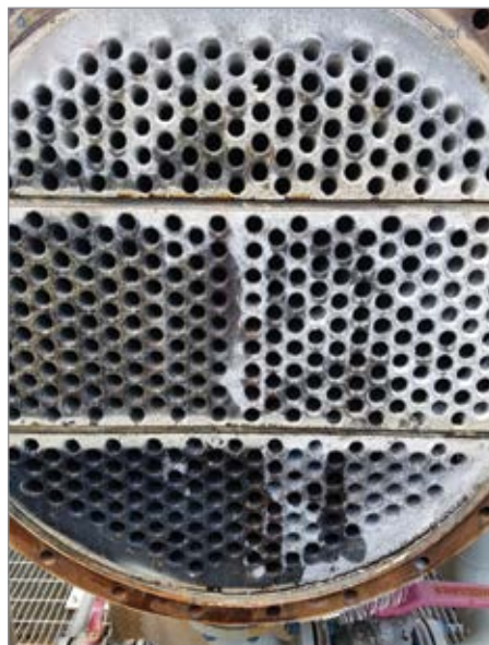
Shown is another heat exchanger at the same chemical plant, which is free of corrosion and scaling when cooling water was treated using FlexPro technology.
