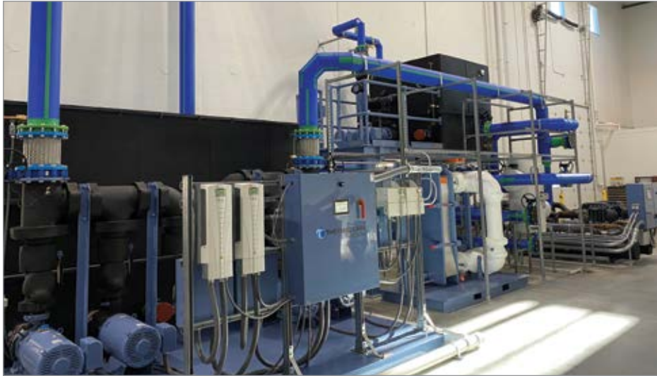
The pump station at SCI's Delavan includes adiabatic fluid cooler and chiller pump tanks for routing chilled water through the process cooling system via Aquatherm Polypropylene (PP-R) piping.
