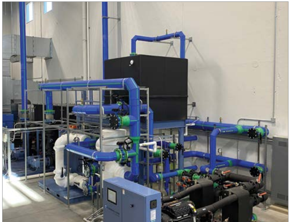
Inside the new SCI production facility is a Thermal Care TCW700 250-ton water-cooled central chiller.
