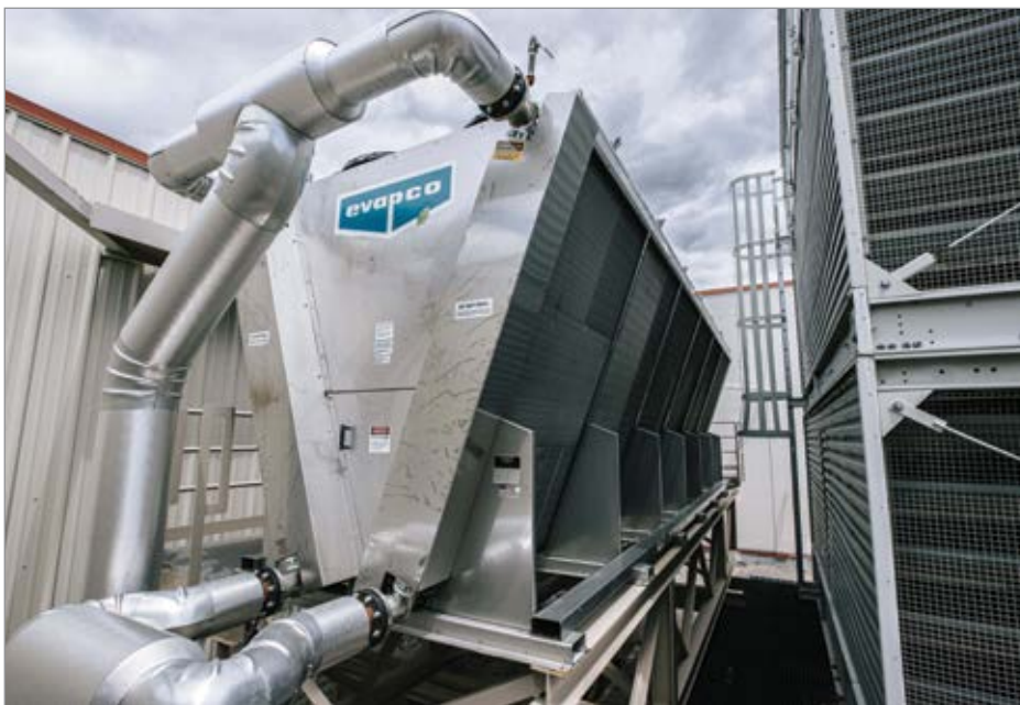
There was just enough room on the roof of the central energy plant at USU’s facility to install the fluid cooler based on existing dunnage.
