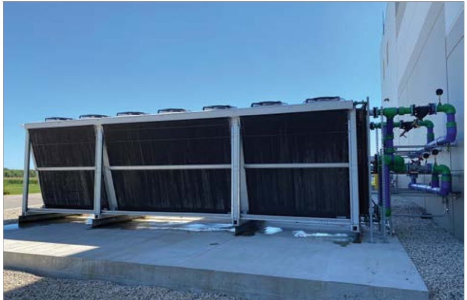
Located outside SCI's new production facility is a Thermal Care HFCG 250-ton, closed-loop adiabatic fluid cooler.
