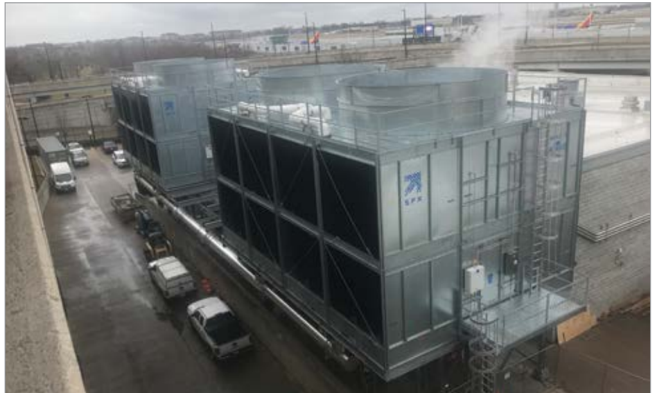
Figure 6. View of New CHRP Cooling Towers from Parking Ramp (courtesy of HMG)
