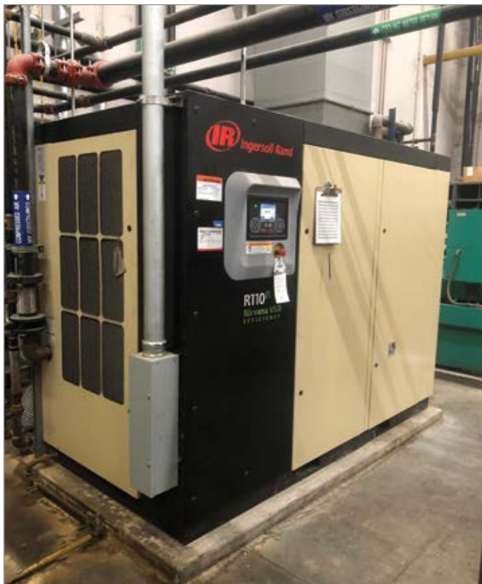
The rotary screw air compressor installed at the Carbondale, Illinois plant.
