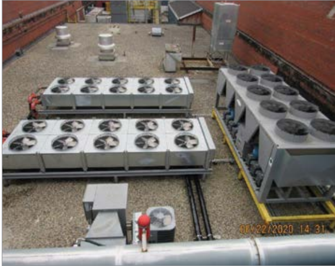
The free-cooling winter cooler installed at the Marysville, Michigan plant.
