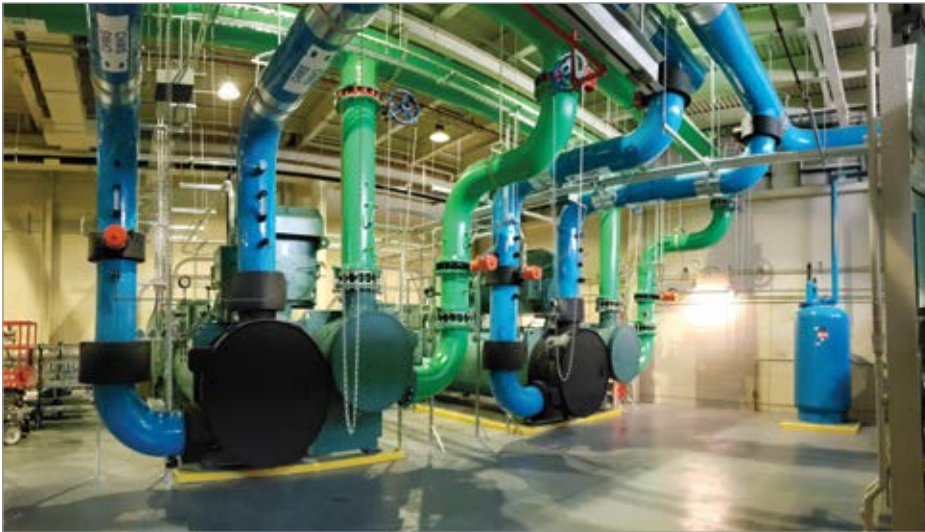
Figure 4. Image of New Lag Chillers
