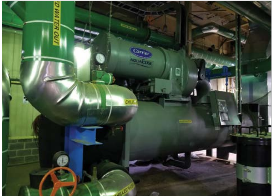
The new 900-ton variable speed chiller.
