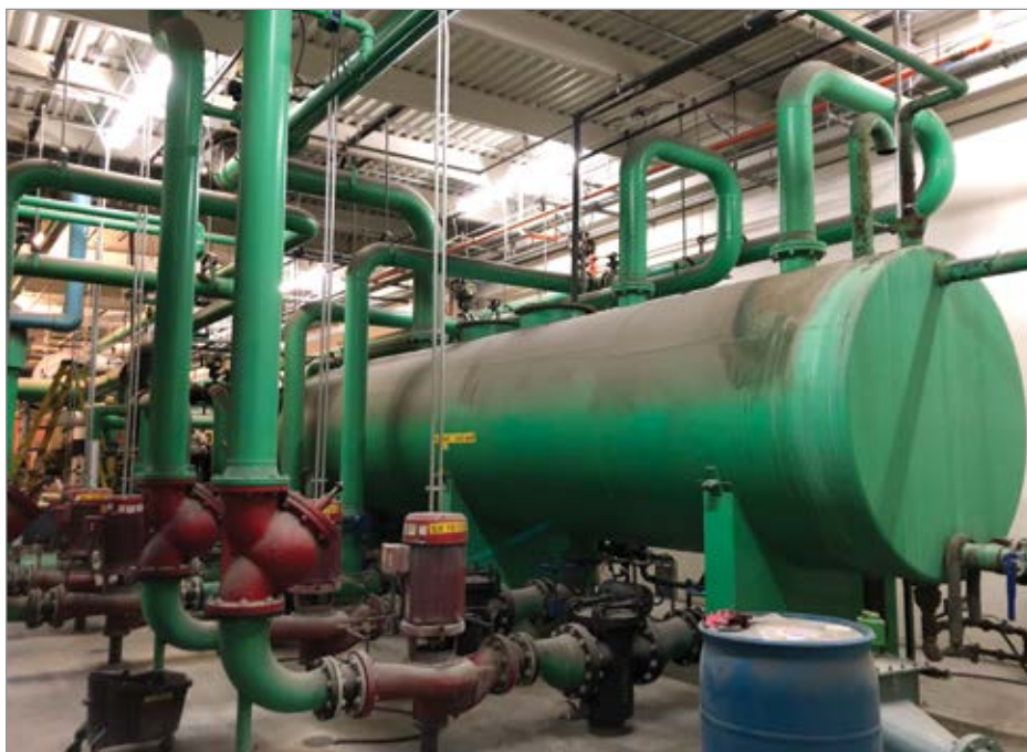
Shown is one of two 10,000-gallon sump tanks used to pre-mix cold and warm cooling water and supply it to the plant’s chillers at 75°F (24°C).
