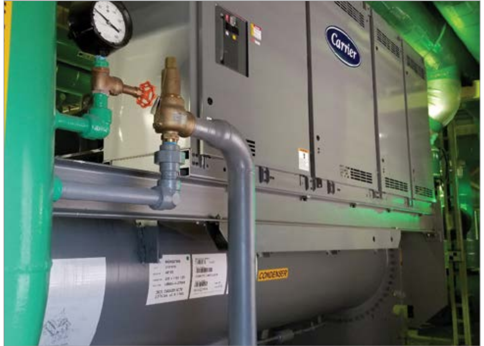
The new 900-ton variable speed chiller.
