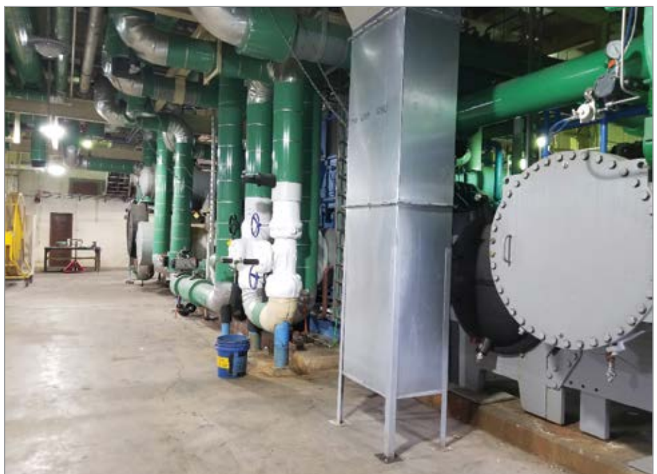
Three chillers provide process chilled water to support the active diffusion process in the plant.
