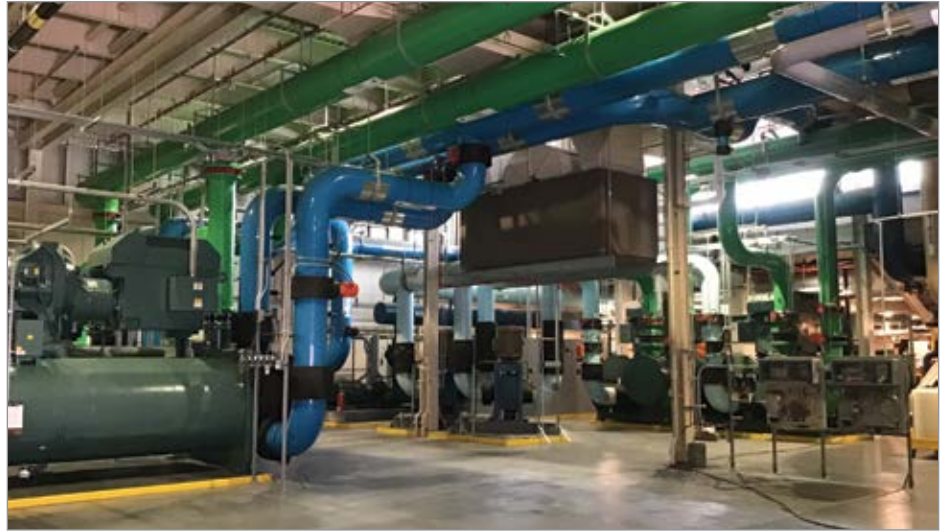
Figure 5. View of New Lag Chillers on Left with Existing Lag Chillers in Center (photo courtesy of HMG)
