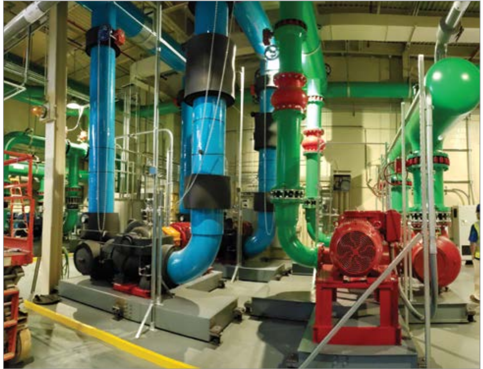
Chilled water and condenser water pumps and 30" condenser water supply pipe.
