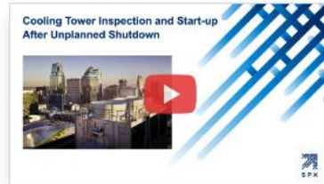
Cooling Tower Inspection and Startup After An Unplanned Shutdown
