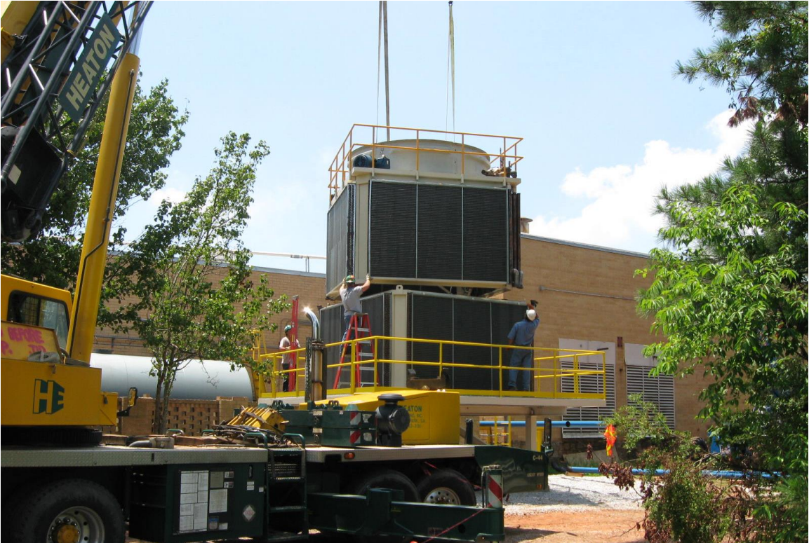
Dry Cooling Tower Erection
